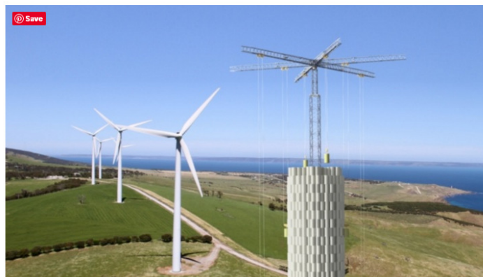
Energy Vault's storage tower consists of a six-crane tower capable of storing 35 MWh. (Courtesy Energy Vault)
